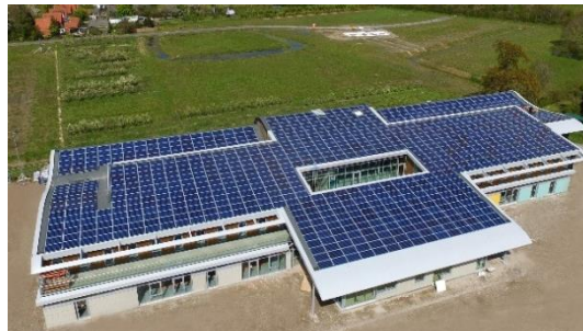
Energie neutrale school Kapelle
